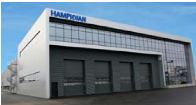
The Hampidjan Group headquarters are located at the waterfront of the main harbor of Reykjavik Iceland in a new 6.500 m2 building.
